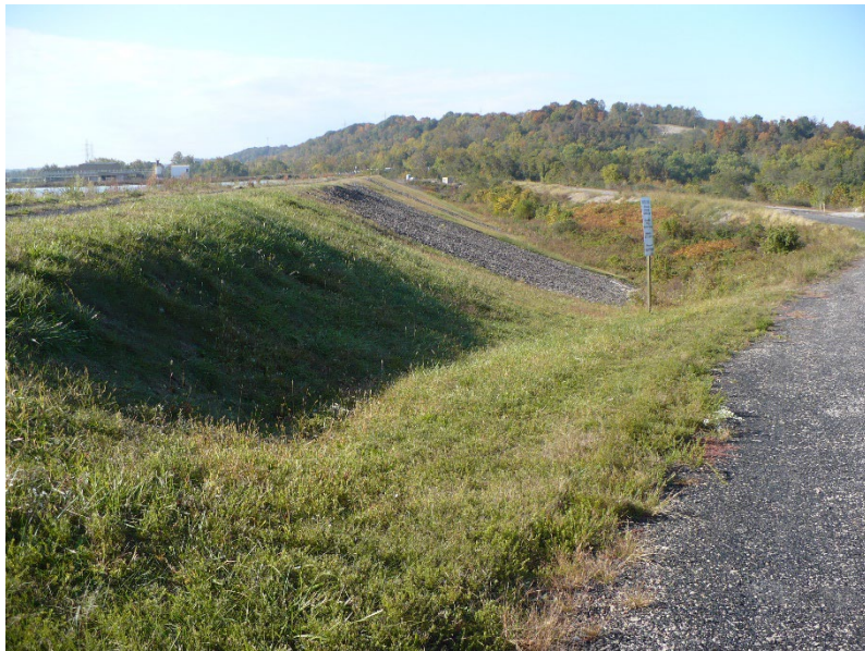
SFAP #3 – exterior slope of west dike-looking south
