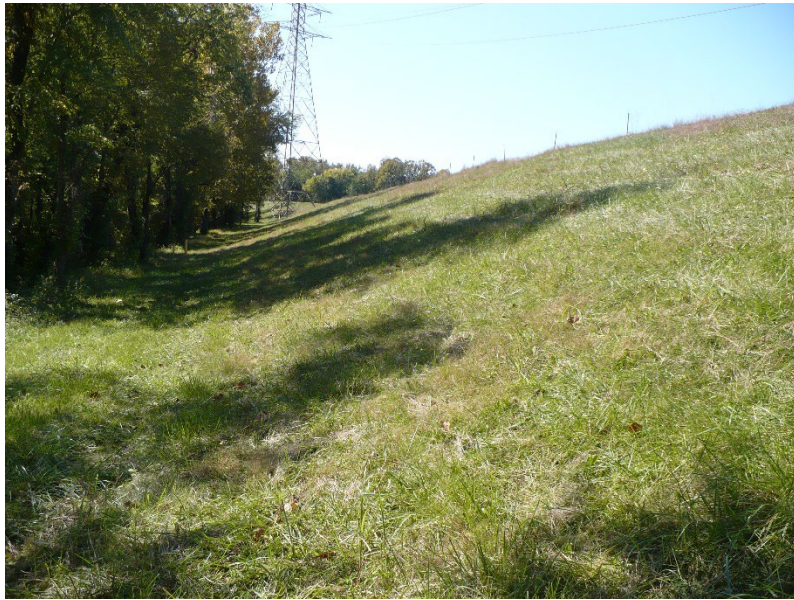
BAP #5 – exterior slope of east dike-looking south
