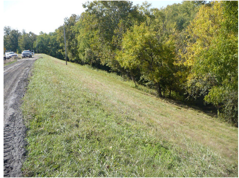
BAP #2 – exterior slope of south dike-looking southeast
