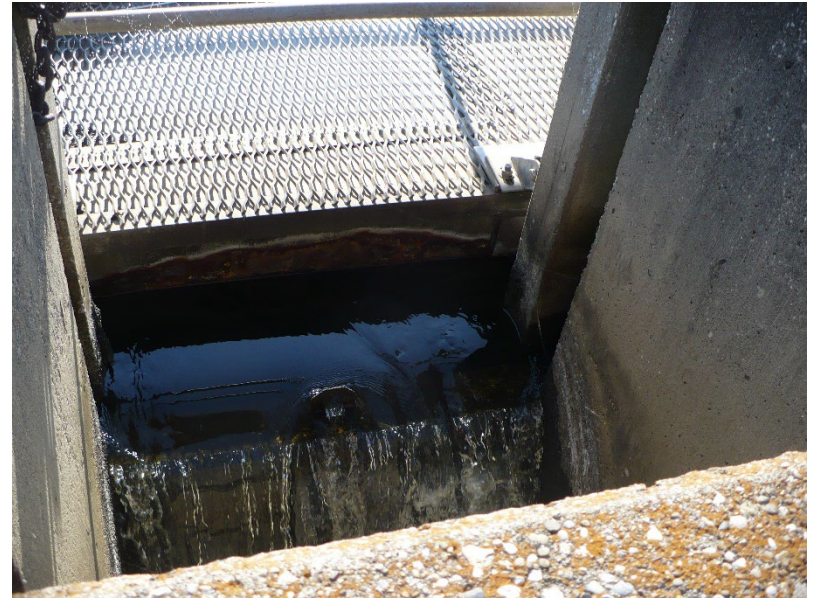
SFAP #6 – outlet structure- smooth flow over stoplog
