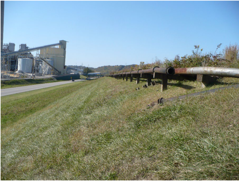
SFAP #5 – exterior slope of east dike-looking south
