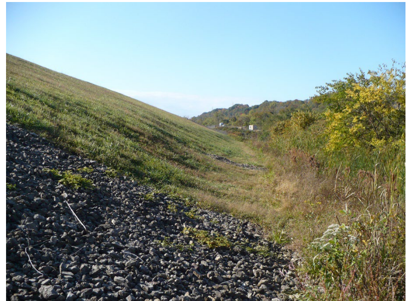
SFAP #4 – exterior slope of west dike-looking south
