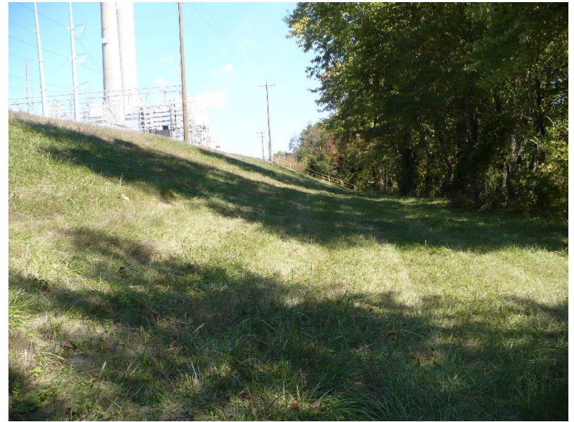
BAP #6 – exterior slope of east dike-looking north
