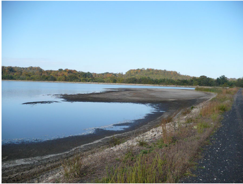
SFAP #1 – interior view of pond
