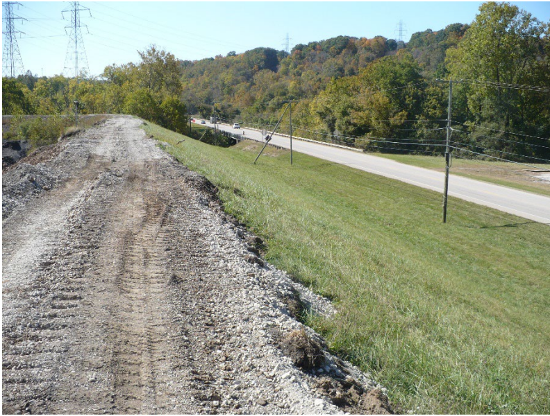
BAP #1 – exterior slope west dike– looking south
