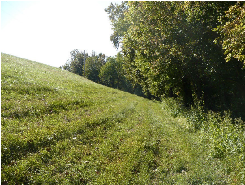
BAP #3 –exterior slope of south dike-looking east
