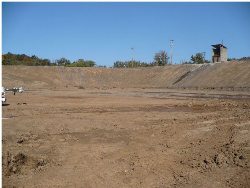
BAP #7 – interior of west portion of BSP
